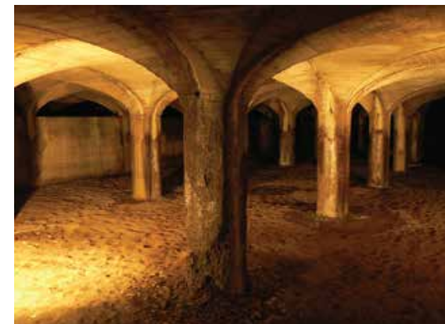
Inglis Falls Conservation Area Water Filtration Plant
