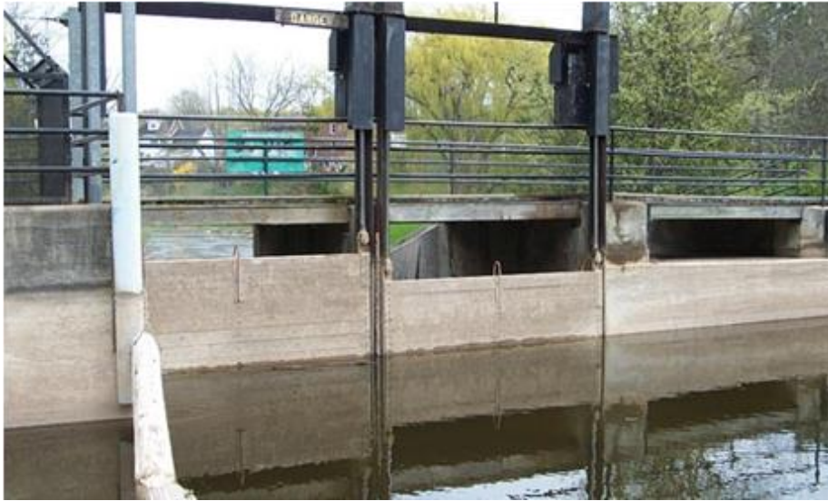
Figure 5 Mill Dam North Gate Setting During Install
