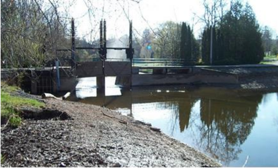
Figure 9 Mill Dam Gate Settings for Draw Down
